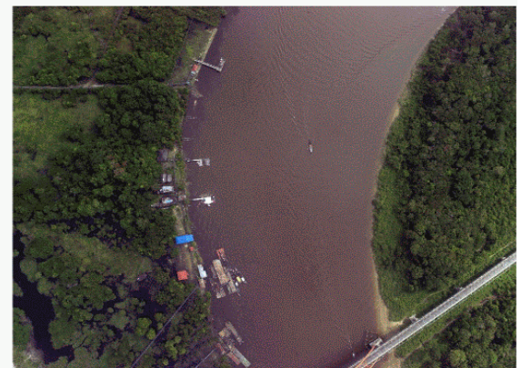
RGB-Ortho-Photo from Kahayan river with bridge in PKY
